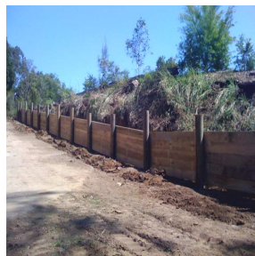
Our new retaining wall!
